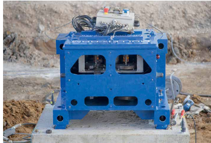
Dynamic excitation of a concrete foundation slab to determine the wave propagation in the soil
