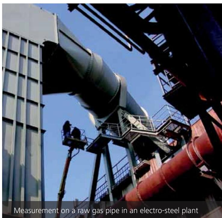
Measurement on a raw gas pipe in an electro-steel plant
