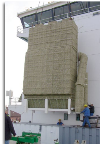
Installation of a desulphurization unit.
